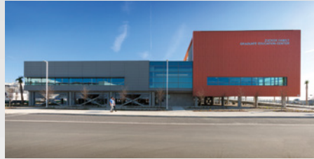
Restoration Institute Graduate Education Center Clemson University LEED-NC, v3.0, 2018 50,000 SF
