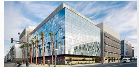
Smith Cardiovascular Research Building University of California San Francisco LEED-NC, v2.2, 2012 232,000 SF
