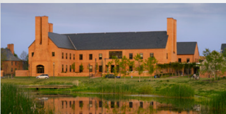
Goodpaster Hall St. Mary's College of Maryland LEED-NC, v2.0, 2008 56,000 SF
