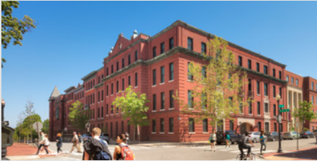
Nevils Hall Renovation Georgetown University LEED-NC, v2.2, 2015 73,535 SF
