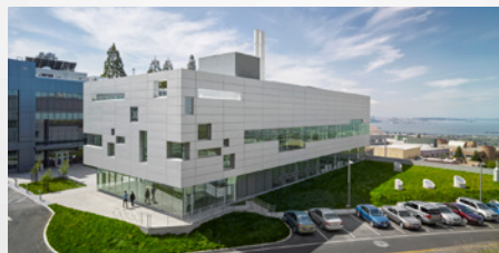
Chu Hall University of California/Lawrence Berkeley National Laboratory LEED-NC, v3.0, 2016 39,000 SF
