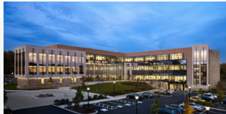
School of Law Villanova University LEED-NC, v2.2, 2010 175,000 SF
