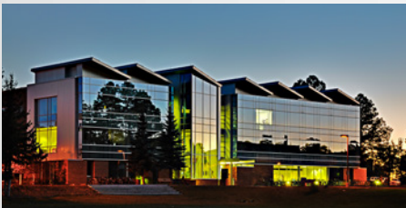
College of Engineering and Natural Sciences Northern Arizona University LEED-NC, v2.1, 2007 90,000 SF
