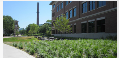
Centennial Hall University of Wisconsin, La Cross LEED-NC, v3.0, 2012 With River Architects 188,570 SF
