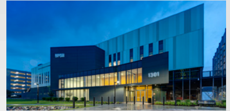
City of Detroit Public Safety Headquarters Detroit Building Authority LEED-NC, v3.0, 2016 400,000 SF
