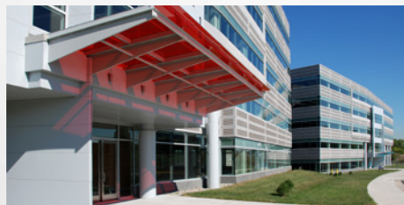
Mission Ridge The Carlyle Group LEED-CS Pilot, 2008 310,000 SF
