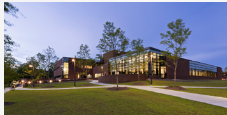
Camp Lejeune Hospital Outpatient Clinic, Naval Hospital Renovation and Addition NAVFAC Mid Atlantic LEED-NC, v2.2, 2014 262,000 SF
