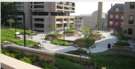
School of Education Renovation University of Wisconsin Madison LEED-NC, v2.2, 2011 With HGA 107,000 SF
