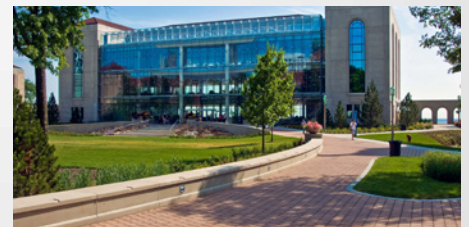
Information Commons Loyola University LEED-NC, v2.1, 2008 With Solomon Cordwell Buenz 69,000 SF
