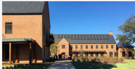
Anne Arundel Hall St. Mary's College of Maryland LEED-NC, v3.0, 2017 39,614 SF
