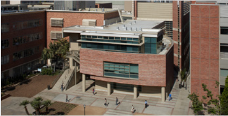
La Kretz Hall University of California Los Angeles LEED-NC, v2.0, 2006 20,000 SF
