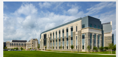
Institute for Critical Technology and Applied Science II Virginia Polytechnic Institute and State University LEED-NC, v2.2, 2011, 42,190 SF
