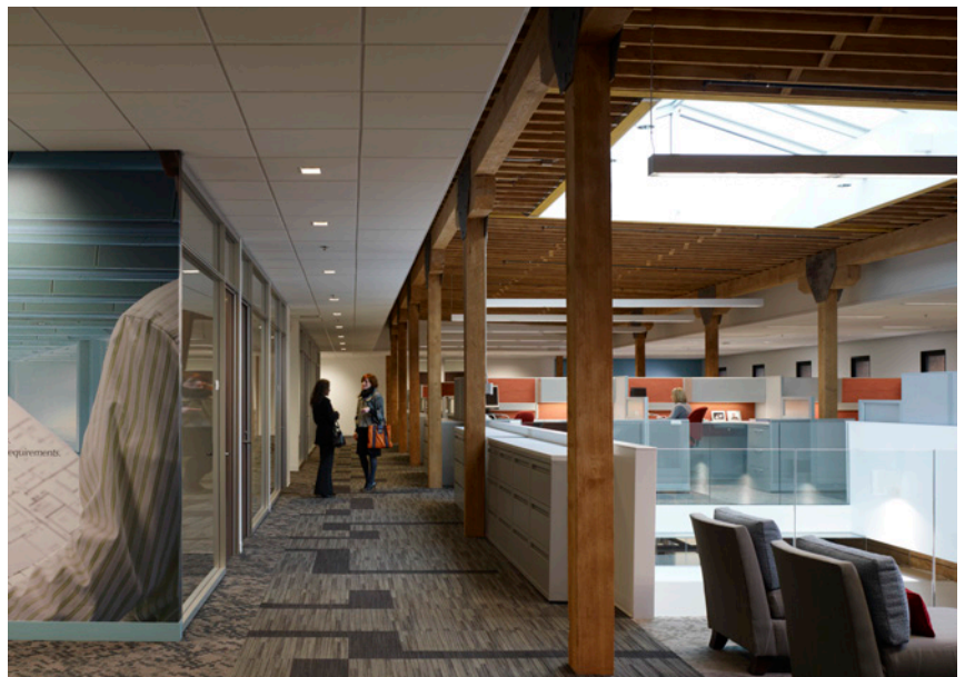
Daylighting for the open office workspace at the HON Company headquarters was achieved by moving private offices from the building’s exterior and opening light wells throughout the existing structure.
